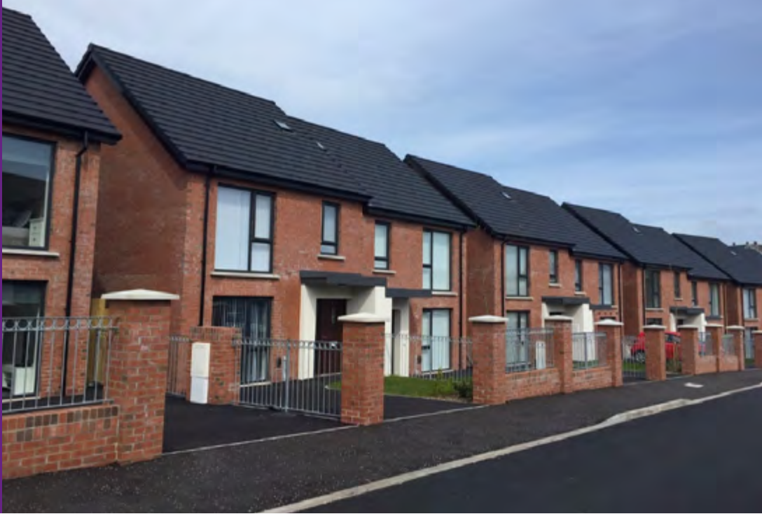
Ballybeen Phase 2 housing (30 social units and two bungalows)
