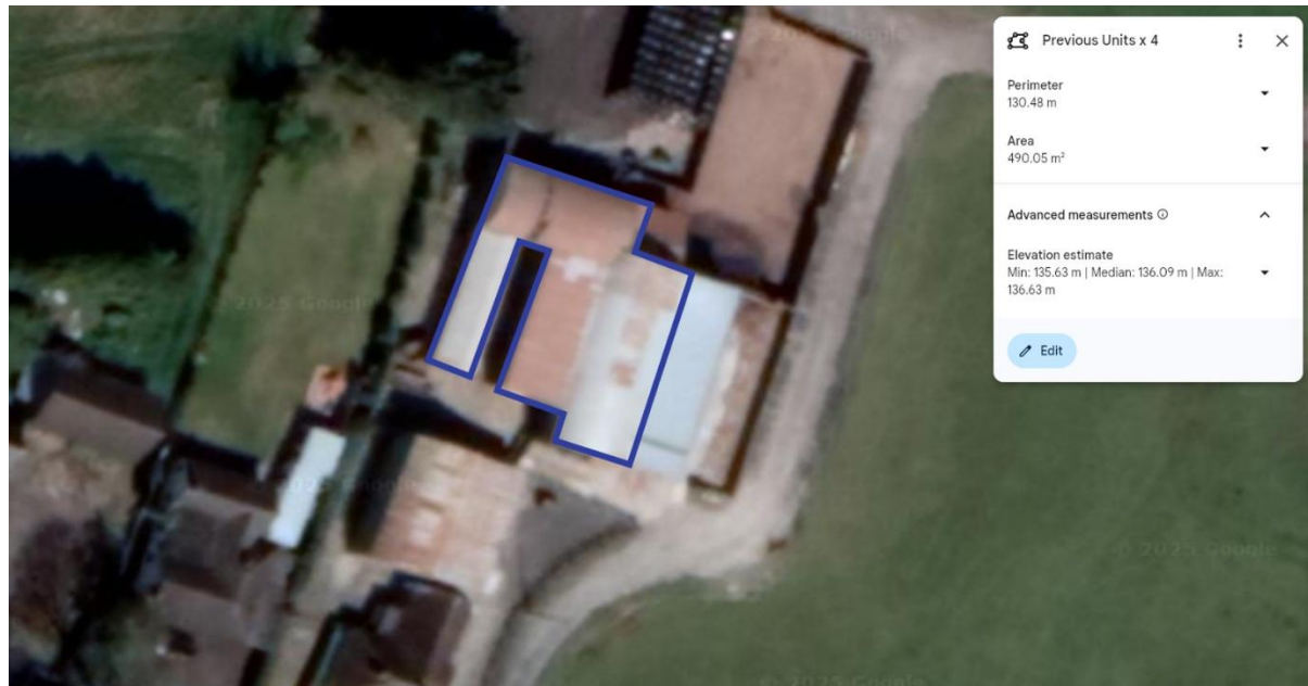
Figure A1: Previous Livestock Sheds – April 2020
